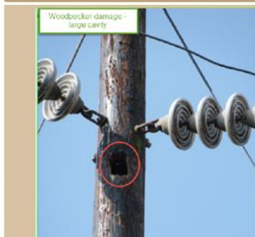
Woodpecker damage - large cavity
