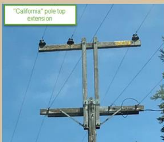
Example: "California" pole top extension
