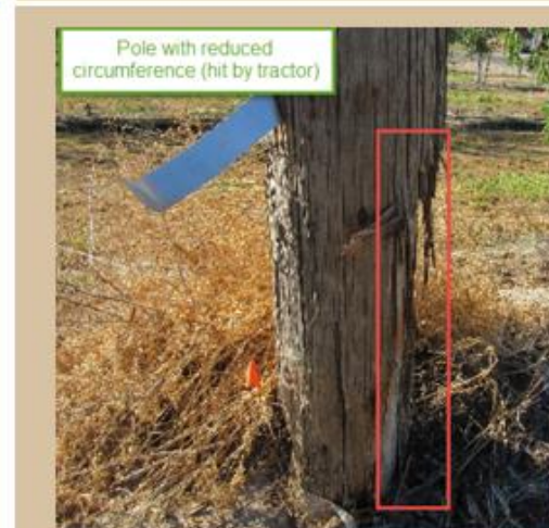
Significant reduced circumference (tractor damage)
