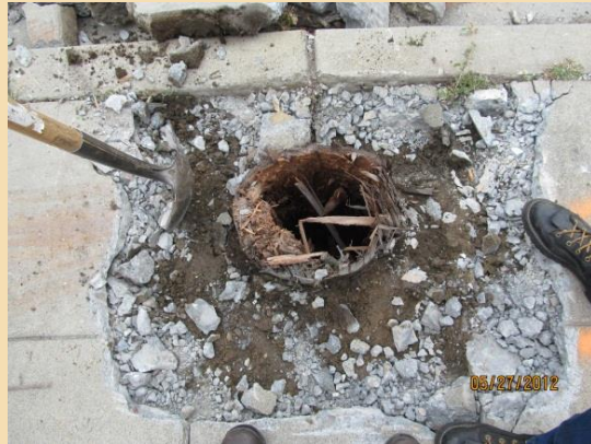
After extraction showing below ground deterioration
