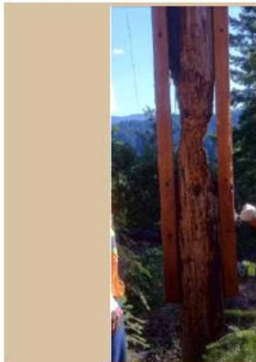
Significant reduced circumference (bear damage)
